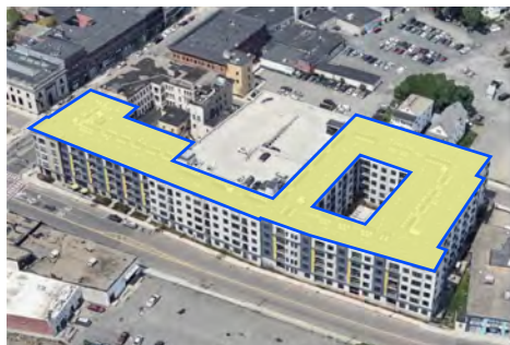
Union House / 45,000 SF (Excluding Garage)
