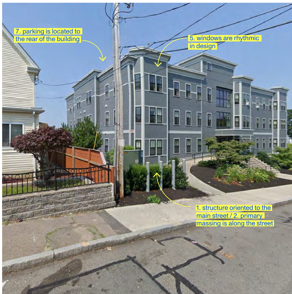
143 Newbury Ave., built in 2019, in relation to Quincy’s design guidelines (image by Google Earth, 2023)
