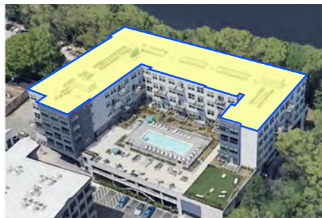
Bancroft Lofts / 26,000 SF (Excluding Garage)
